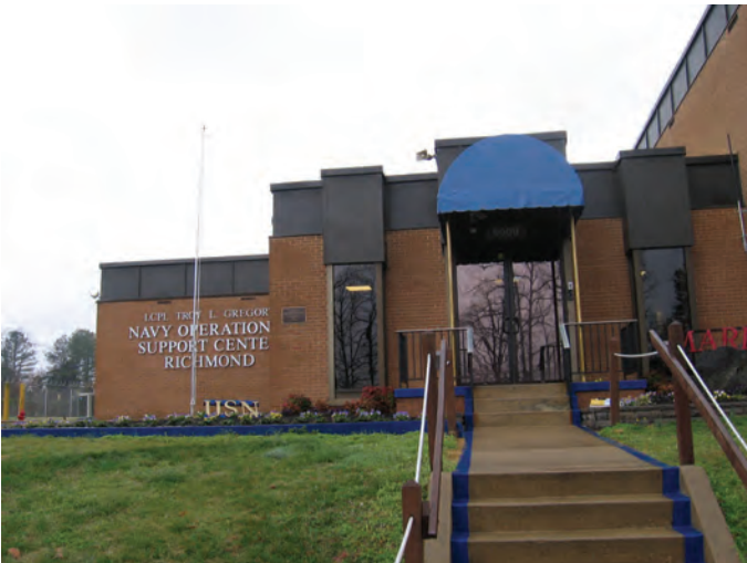
Navy Operation Support Center—Richmond.
